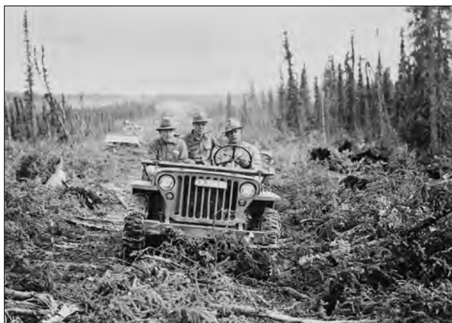
This Army jeep was the first truck to travel over the rough corduroy road on the Alcan (the Alaska Highway). Corduroy road is made by placing logs, branches, or boards side by side across a roadway that's swampy or muddy. Photo retrieved from the Library of Congress
