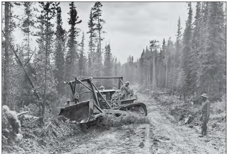
A Caterpillar tractor with a grader widens the road on the Alcan (the Alaska Highway) in 1942. Photo retrieved from the Library of Congress
