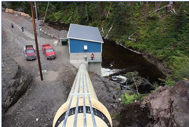
The Gartina Falls Hydroelectric run-of-river system near Hoonah currently provides 25-30 percent of the city's power, on average. Photo by the National Oceanic and Atmospheric Administration.
